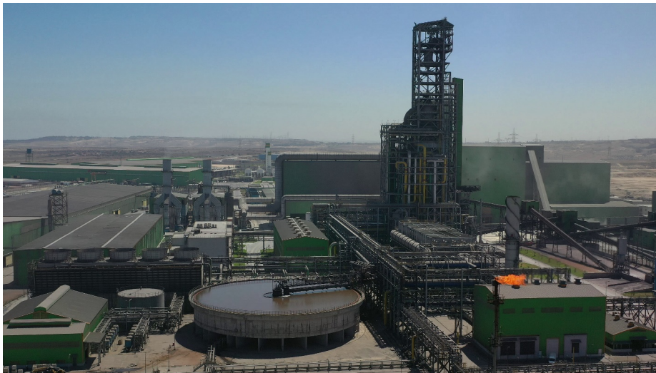
Tosyali Algeria Integrated DRI-EAF Steel Mill in Bethioua (Oran), Algeria
