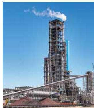
voestalpine Texas HBI Plant
