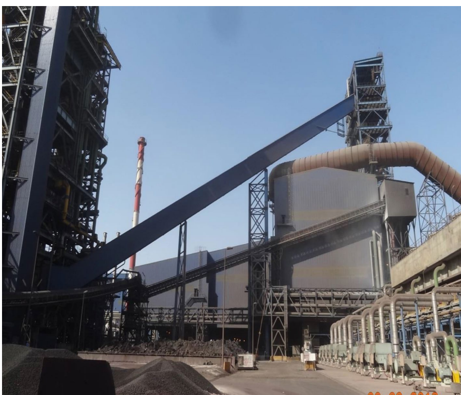
FIGURE 3 Hot DRI transport conveyor from the MIDREX® Shaft Furnace to the melt shop
