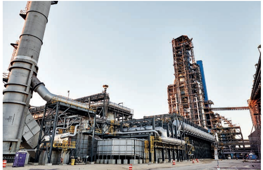
MIDREX HBI PLANT: CORPUS CHRISTI, TEXAS, U.S.A.
