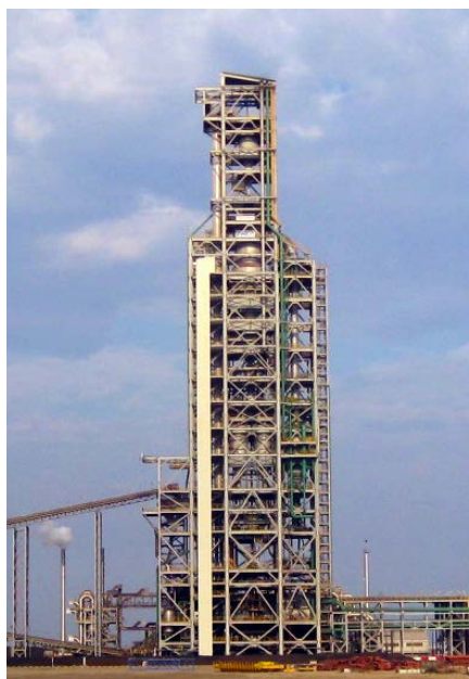
Jindal Steel Sohar HOTLINK Shaft Furnace (Height: 148 m)
