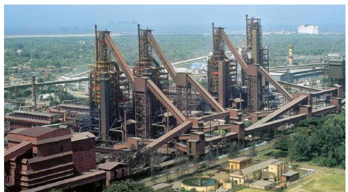
ArcelorMittal/Nippon Steel India
