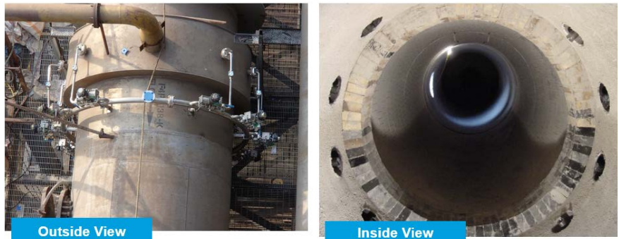
FIGURE 5. Reformer Gas Mixer- Outside / Inside Views
