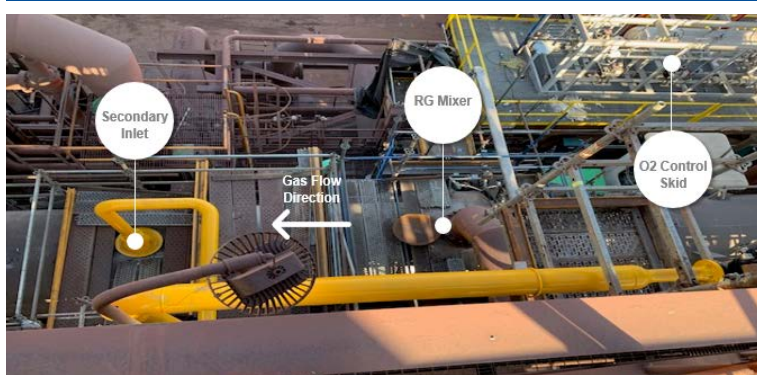
FIGURE 9. Secondary enrichment natural gas inlet nozzle
