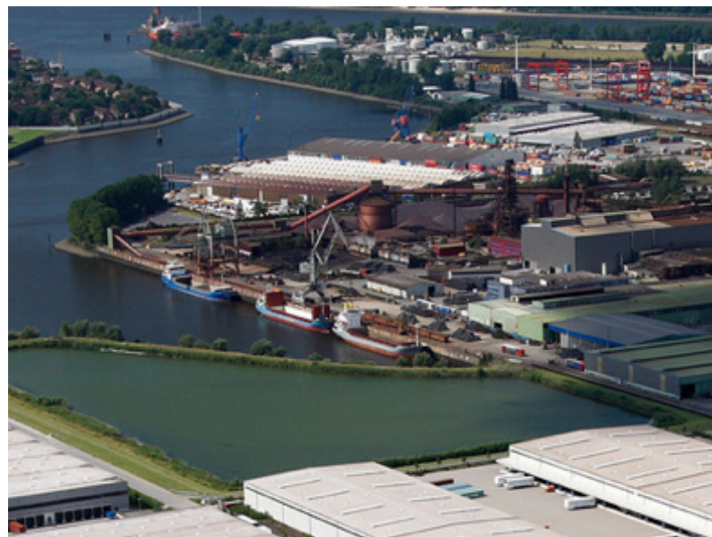
FIGURE 6. MIDREX Plant Owned and Operated by ArcelorMittal
