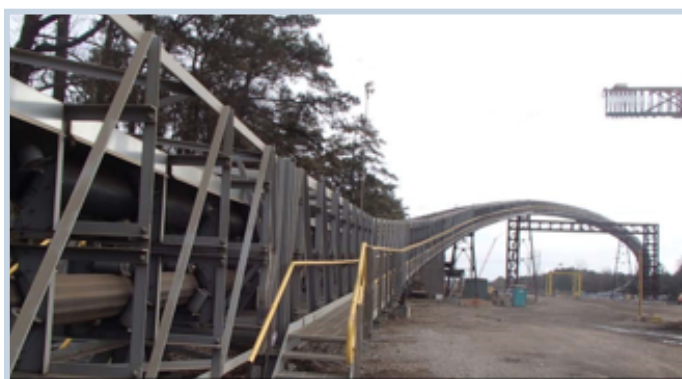
FIGURE 2. Pipe Belt Conveyor Carrying CDRI [3]
