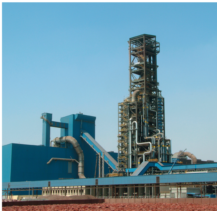
Hadeed Module E, Hot Transport Conveyor and EAF Meltshop.
