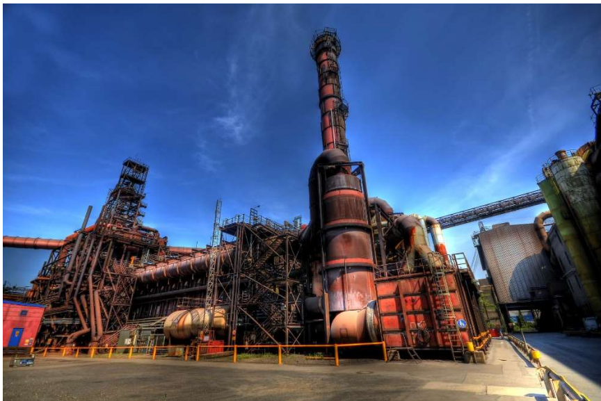
The existing Midrex plant at the Hamburg production site is the one with the lowest CO 2 -emissions for high quality steel production in Europe. It processes about 980,000 tons of iron ore pellets a year, making it an iron sponge, which is 95 percent metallic iron. Photos: ArcelorMittal
