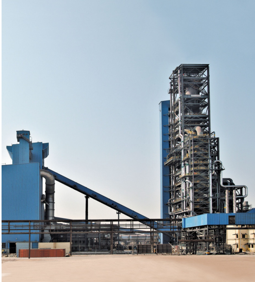
Figure 4 Hot Transport Conveyor at HADEED Module E
