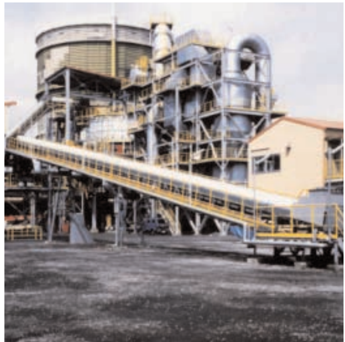
Figure 6 - Hirohata FASTMET Plant
