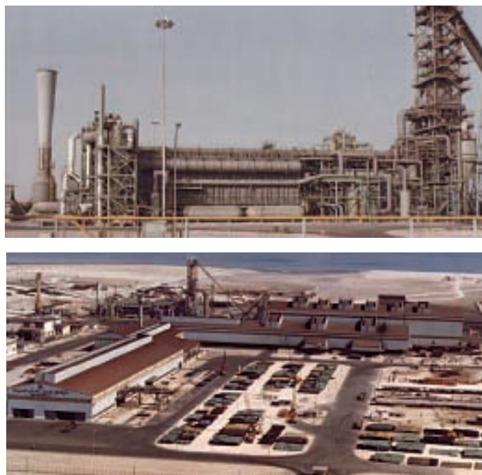
Figure 3 - QATAR Steel Company
