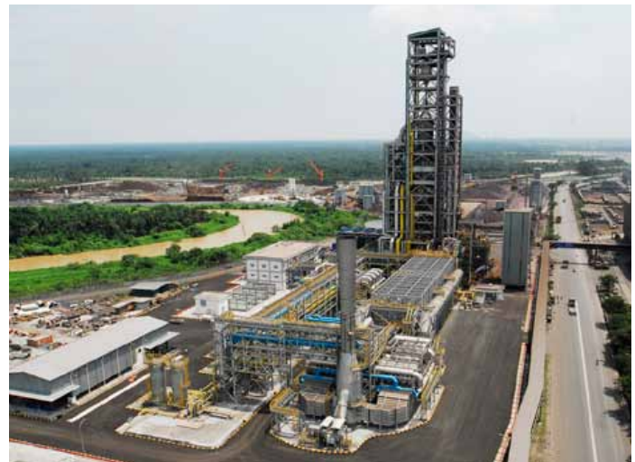
FIGURE 1 LION'S MIDREX Plant in Banting, Malaysia
