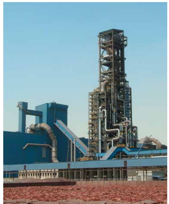
FIGURE 4 Hadeed Module E, Hot Transport Conveyor and Meltshop
