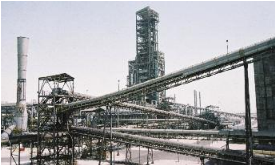
Figure 2 - Qatar Steel: DRI-2 MIDREX Plant
