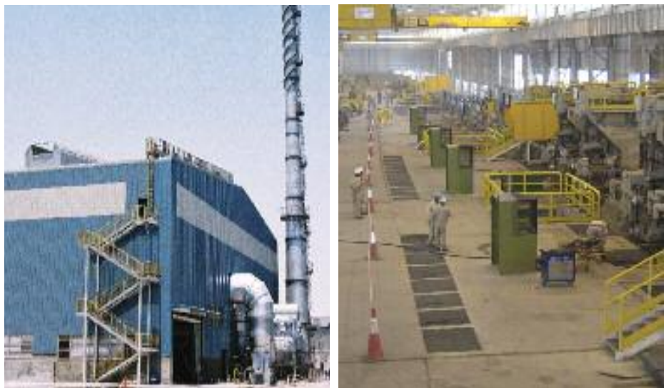
Figure 6 - Qatar Steel: View of New Rolling Mill (RM2) Building and Shop
