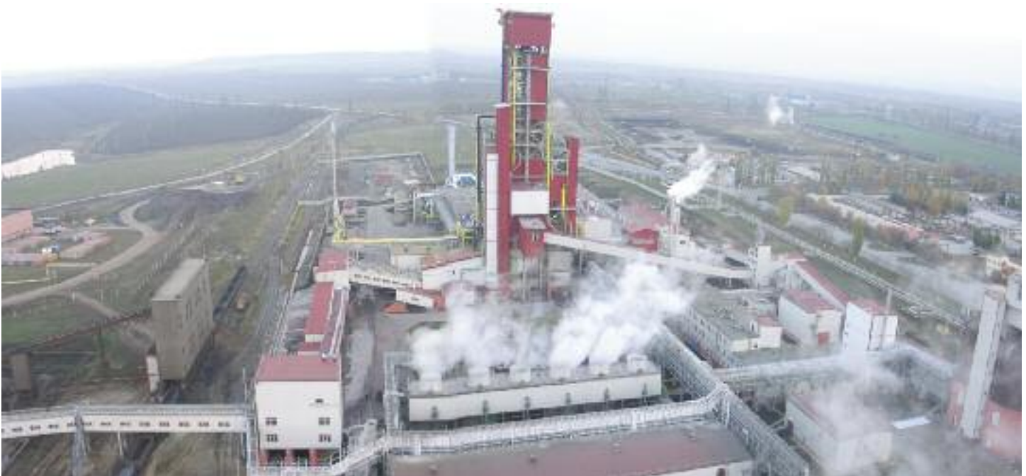
Figure 4 - LGOK MIDREX Plant
