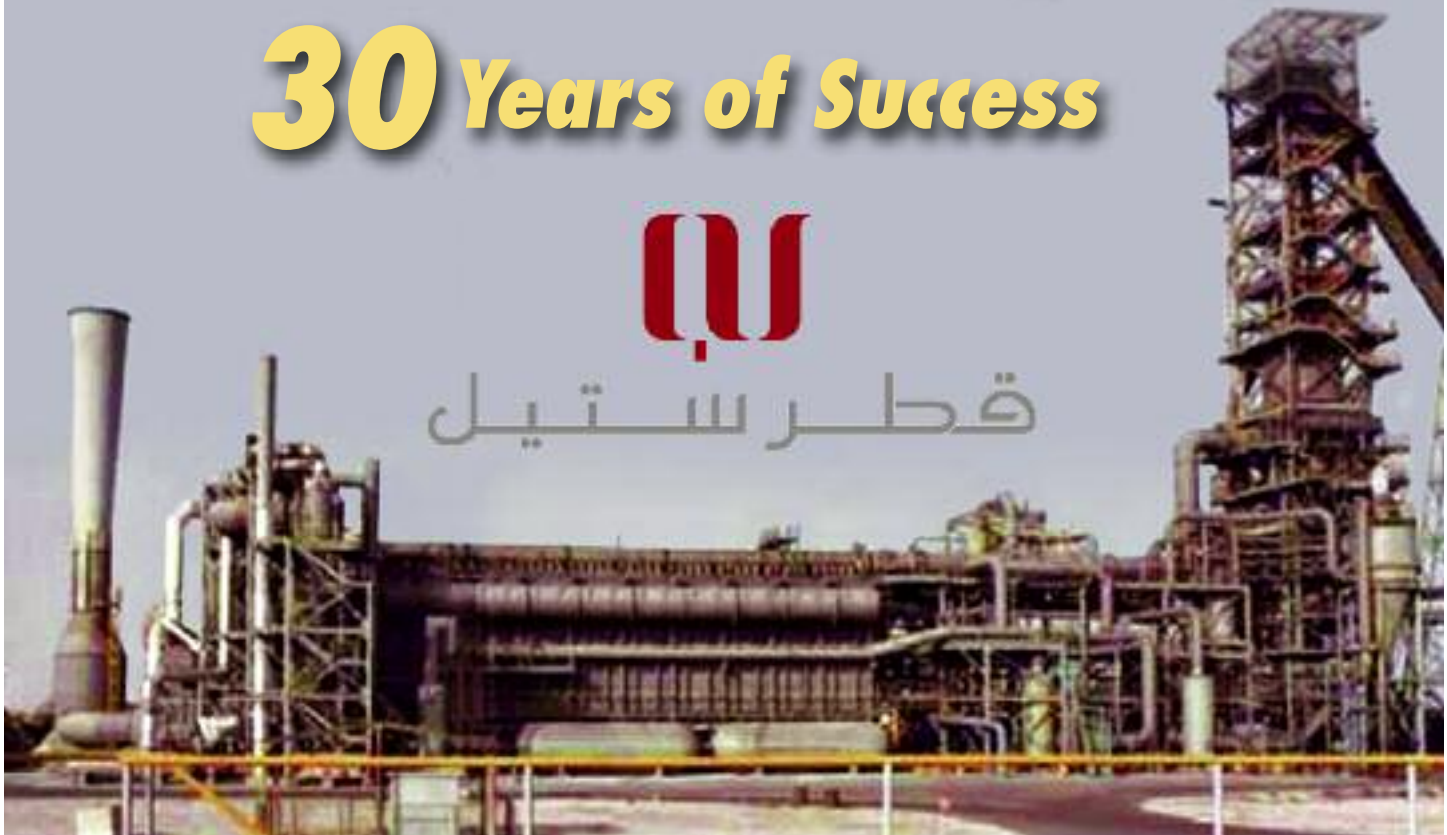
Figure 1 - Qatar Steel: DRI-1 MIDREX Plant
