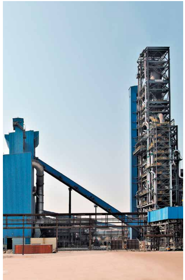
FIGURE 4 MIDREX Plant at Hadeed, Saudi Arabia Including Hot Transport Conveyor System
