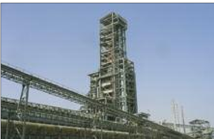
Qatar Steel Company Module 2
