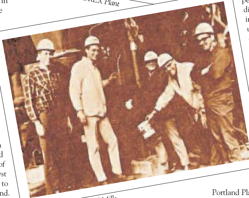
First DRI at Oregon Steel Mills
