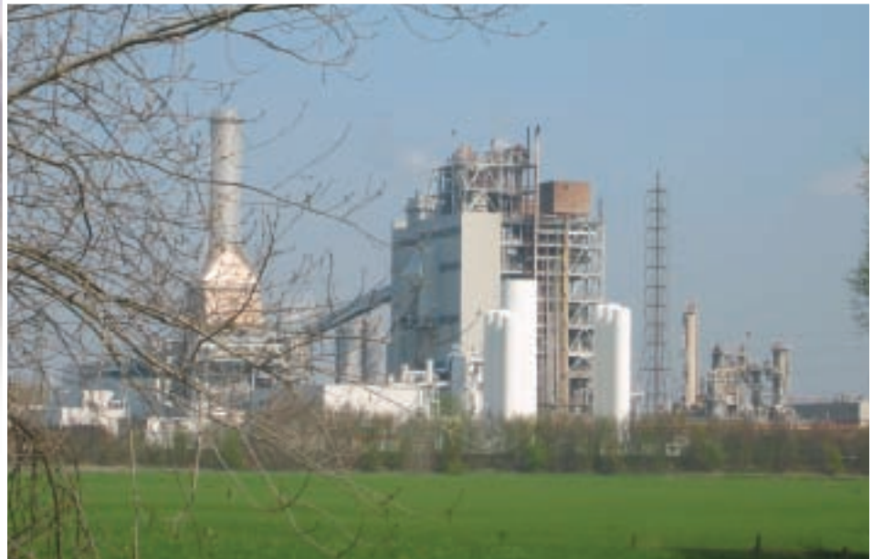
Shell Gasification Plant Buggenum, Netherlands
