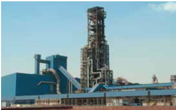
FIGURE 4 Hadeed MIDREX Plant
